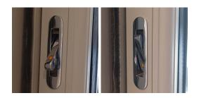
If your window has restrictors, push the restrictor inward to override the mechanism. (restrictors approximately 100mm)
