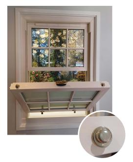
Use the lift hooks to lift the bottom sash slightly. Do not attempt to tilt the sash if it's been lifted all the way to the top.
