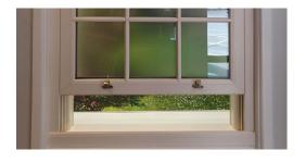
Push the bottom sash upwards. To close, simply push the sash down until you hear a click signalling the sash is in place.
