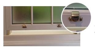
Use lift hooks to open the bottom sash slightly. Push from the centre or with equal force on both sides if your window is not fitted with lift hooks.
