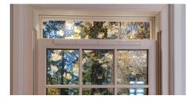
Once the bottom sash has been pulled upwards slightly, you can then pull the top sash down.
