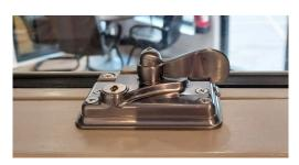
To operate the sash window, start by unlocking the sashes. Simply lock and unlock the sashes by turning the lever side to side.
