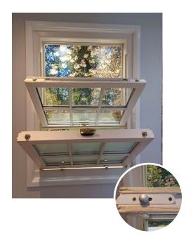
To tilt the top sash, the bottom sash must already be tilted. Pull the top sash down.
