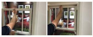
Step 3 - Keeping the sash level, push the bottom sash back into the frame fully. You will again hear a 'click' as it engages back in to the frame.
