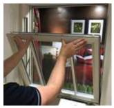
Step 2 - Slide the top sash back up to the top of the frame.
