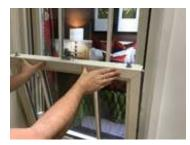
Step 4 - Once the bottom back slide the sash down the sill.
