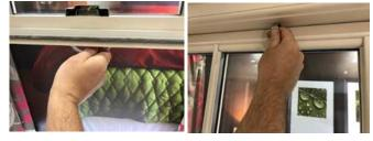
Step 6 - On the top of the sash locate the tilt catches and slide both at the same time towards the middle of the sash the same way the bottom sash buttons operate.
