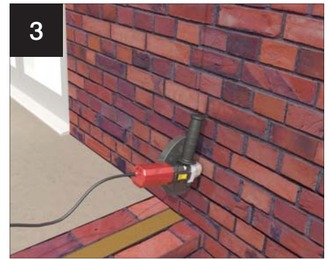
3 Mark and grind out brickwork for vertical DPC
