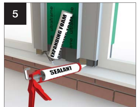
Weatherseal any joints/gaps under column and between windows/doors and columns. Use foam and/or appropriate sealant.
