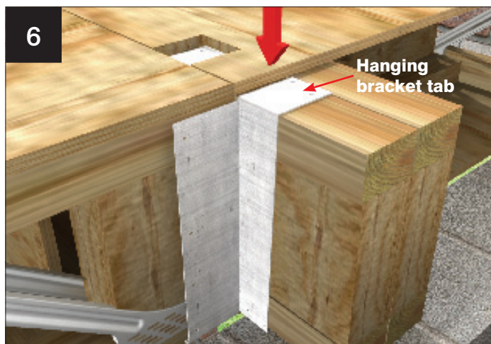
From the top, tap down the hanging bracket tab and secure in place using 65mm round head nails.
