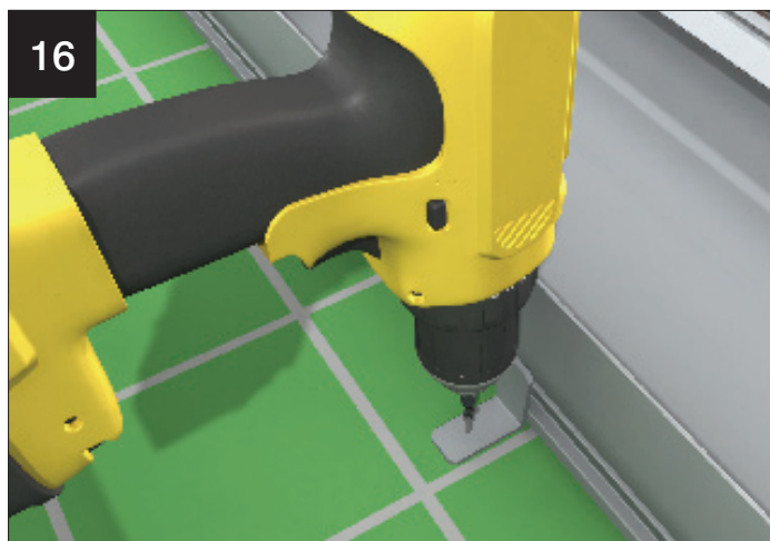
Screw fix the box gutter down to the structural cassette using the brackets supplied.
