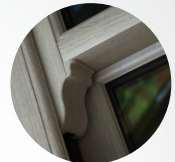
Run-through Sash Horns
