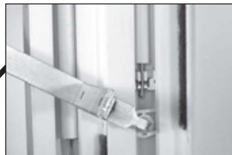
Access to the balance is now gained - repeat steps 2 & 3 of the bottom sash procedure.
