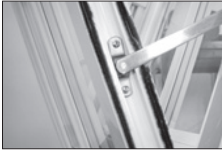
Fig 1 Remove screws from both sides of the sash
