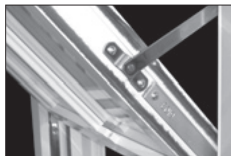
Fig 7 Fig 8 Remove all screws from both sides of the sash
