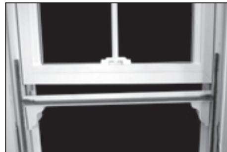
Fig 6 Remove sash interlock
